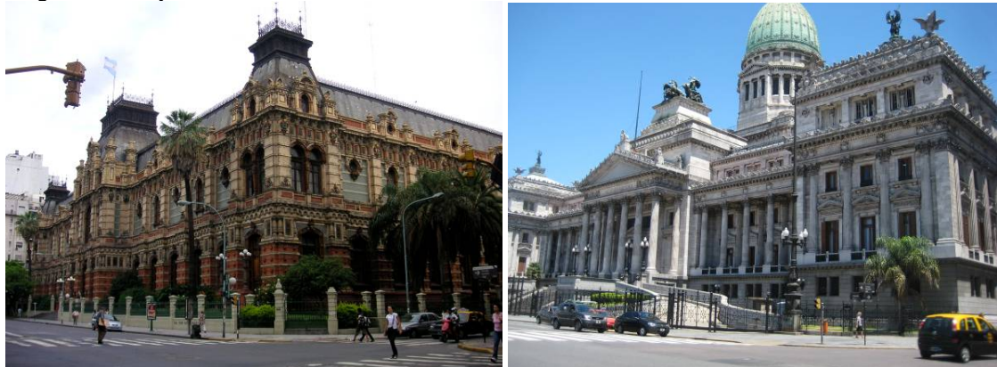
There is some wonderful architecture in both Buenos Aires and Montevideo - Left: The Palacio de Aguas Corrientes – a grand Victorian edifice, built to house a water pumping station. The exterior terra cotta tiles came from the Doulton and Burmantofts factories. Right: The Palacio del Congreso – the parliament buildings for the Government of Argentina.
